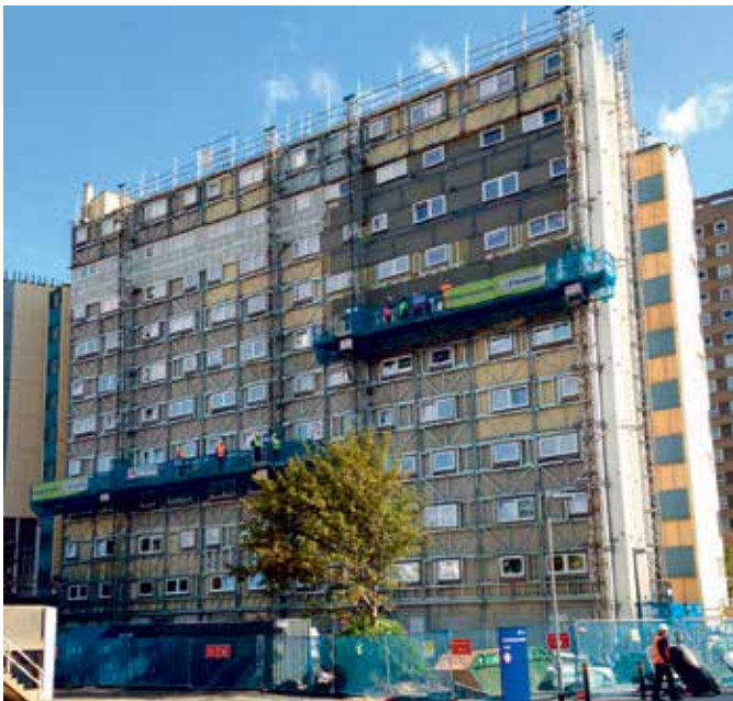
Retrofitting the 11-storey residential block, Wilmcote House in Portsmouth, UK, with use of external wall insulation means residents can occupy the building while the construction is going on.
