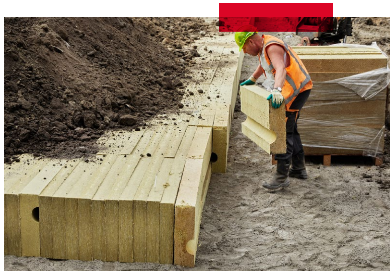
Manually installing 500mm high Rockflow elements.
