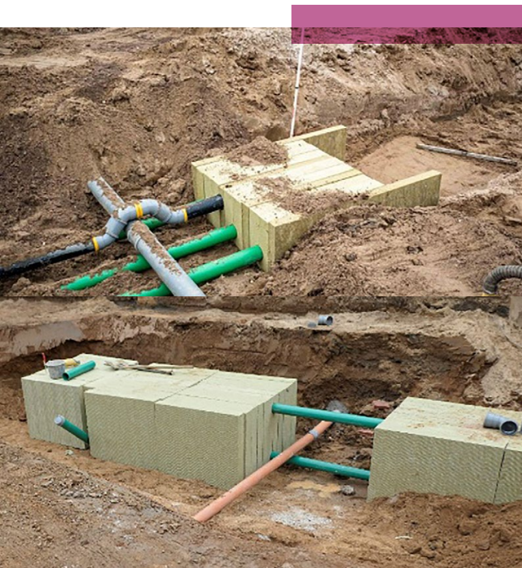
Ducts or pipes as obstacles. In a linear attenuation and infiltration system, the stone wool may be interrupted and connected to the next stone wool element with an appropriate pipe. This makes it unnecessary to move existing services and avoids delays on site or inconvenience for local residents or businesses.
