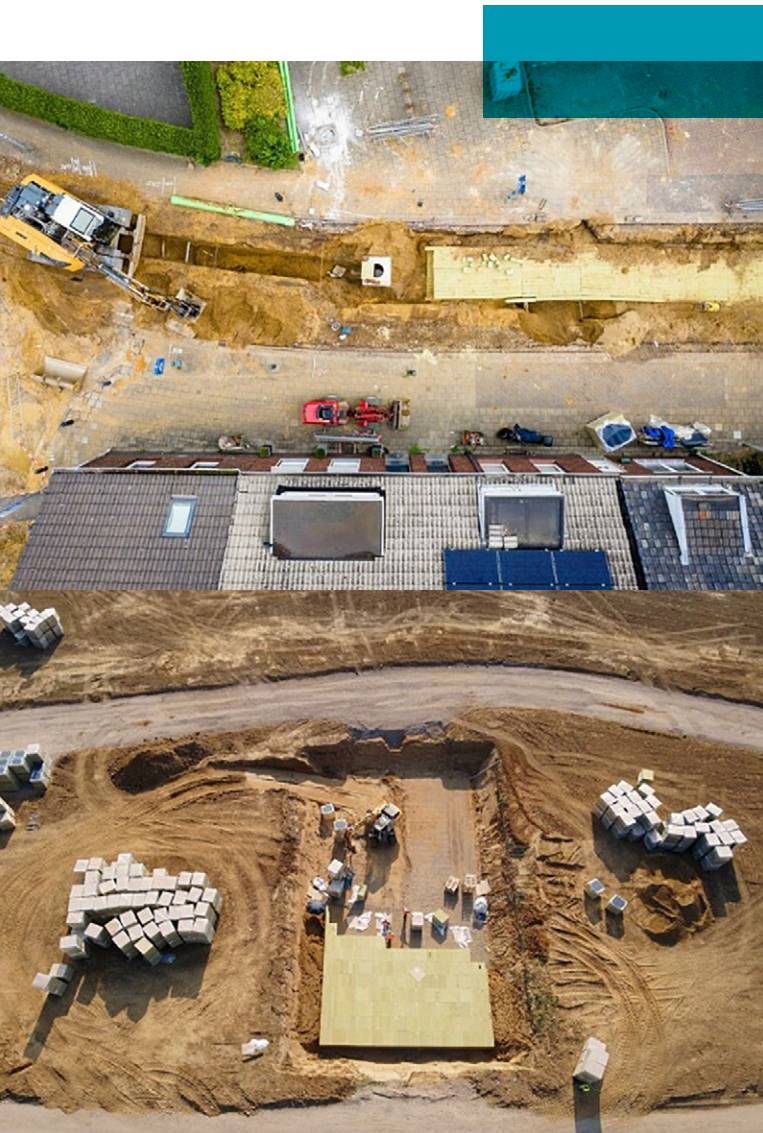
Rockflow installed as linear infiltration (top) or a central attenuation and infiltration system (above).
