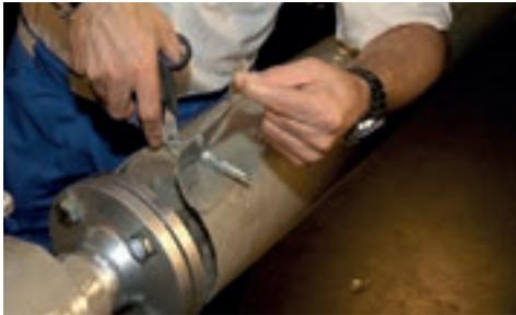
ProRox® GRP 1000 can be cut or trimmed into any shape.
