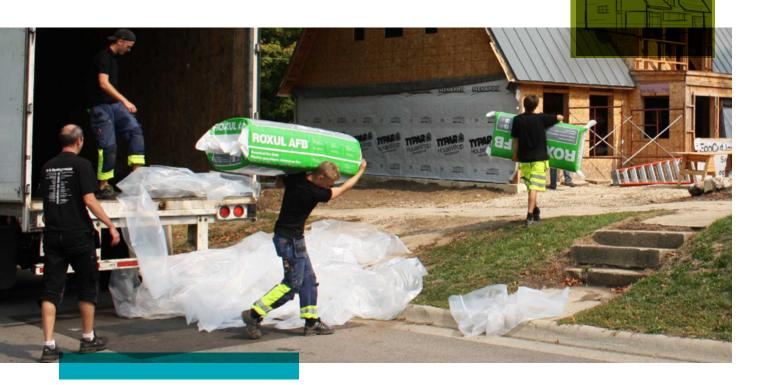
Layering. That is the key to the Scandinavian principle of residential construction. The idea that layering insulation in different stages within the wall assembly eliminates thermal bridging and creates an energy efficient, continuously insulated, air-tight envelope has been part of building practices in Sweden and other parts of Scandinavia for years.
