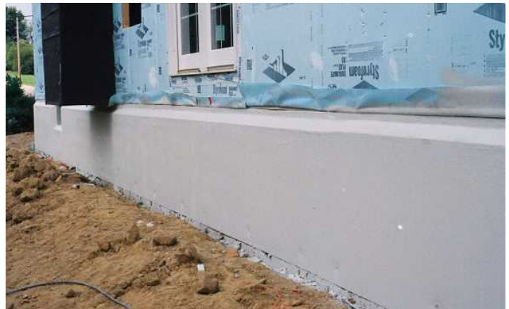
Photo 1 Stucco as Protection - It has impact limitations
