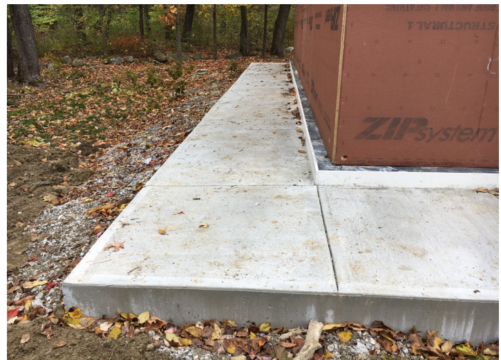
Photo 7 Concrete Skirt – Protecting rigid horizontal insulation
