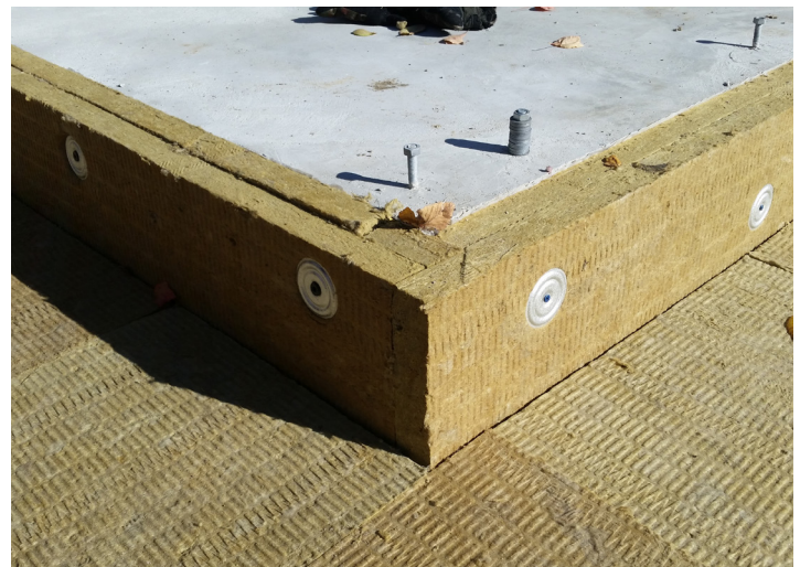
Photo 6 Shallow Frost Protected Foundation – Rigid horizontal insulation
