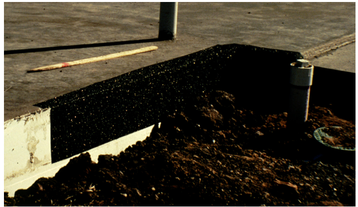
Photo 2 Fully Adhered Membrane - "Roofing" strip used to protect slab edge insulation
