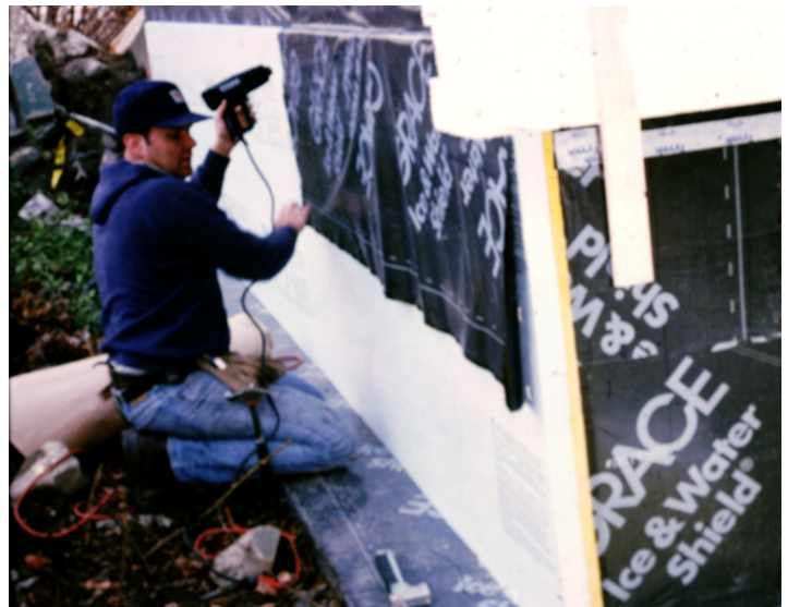
Photo 3 Aluminum Sheet – Rigid insulation with a membrane seal prior to installation of the aluminum
