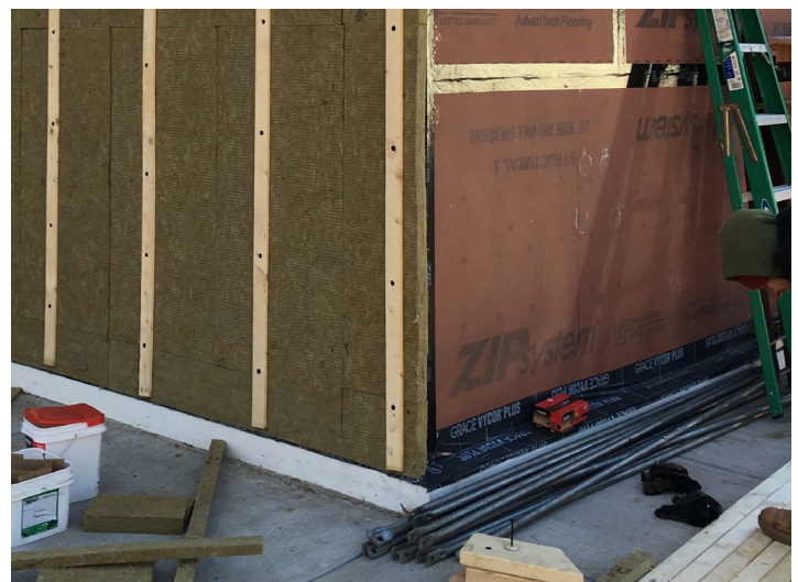
Photo 8 Cellular PVC - Fully adhered membrane and a strip of aluminum or alternatively a strip of cellular PVC protecting the insulation.
