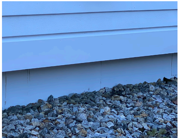
Photo 4 Aluminum Sheet – Completed installation
