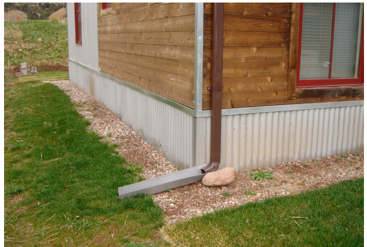
Photo 5 Rigid Metal Sheetting - Exterior foundation insulation is protected by rigid metal sheeting
