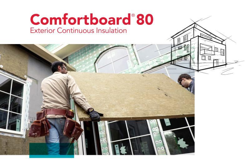
ROCKWOOL Comfortboard<sup>®</sup> 80 thermal insulated sheathing is a rigid stone wool insulation board designed for use as an exterior continuous insulation. Comfortboard<sup>®</sup> 80 does not produce smoke or propagate flames, keeping occupants safe and reducing property damage in the event of a fire. Vapor permeable, this solution allows fast outward drying, keeping moisture out of your wall assembly.
