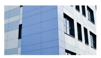
Rockpanel Premium A2 boards fulfil the highest European fire protection standard and secure a flawless façade design with no visible rivets or screws.
