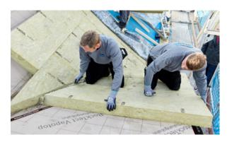
A ROCKWOOL weatherproof vapour barrier was installed to ensure the roof was initially protected, followed by the ROCKWOOL fire-safe insulation solution for pitched roofs.
