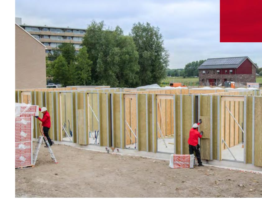
The key element of the Rockzero concept is a load-bearing stone wool column reinforced with steel. The Rockzero column contains a total of 3 zones; a structural zone in the centre, a service void for electric and plumber installations on the inside and the main insulation zone on the outside.
