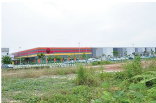
First Solar photovoltaic plant, Kulim, Malaysia
