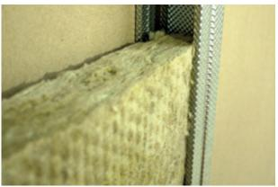
It is also simple to cut Safe 'n' Silent Pro to size with a serrated knife, for a fast and easy installation between studs, around electrical boxes, pipes, wiring, ductwork and even between studs and joists of non-standard widths.
