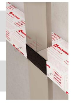
2. The intumescent strip should be continuous over the rail and secured either side with pigtail screws.
