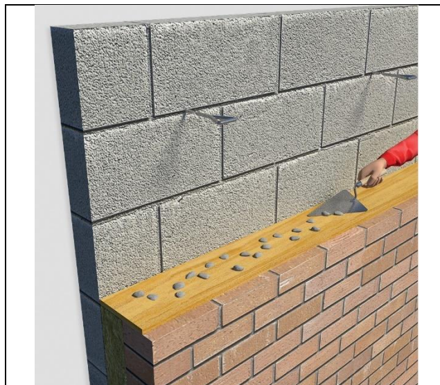
Figure 2 Use of a cavity board when clearing off mortar
