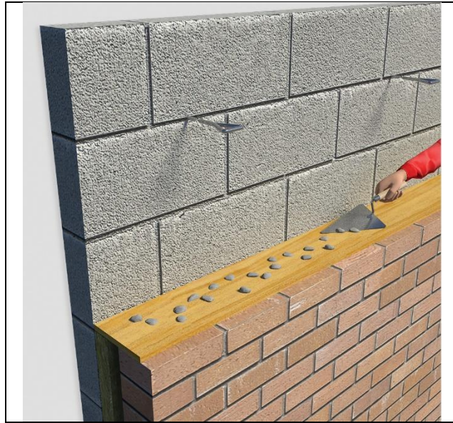
Figure 2 Use of a cavity board when clearing off mortar
