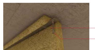
50mm Fire Barrier compressed between soffit and clamping plate at max 450mm centres
