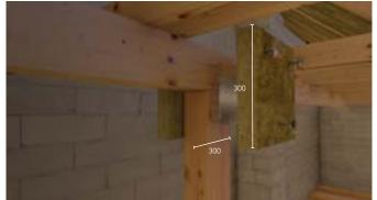
25mm thick ROCKWOOL BeamClad® fixed with FirePro Glue and nailed, or 50mm Fire Barrier secured with screws and large square washers. Use 50mm nails for BeamClad and 70mm screws for Fire Barrier.
