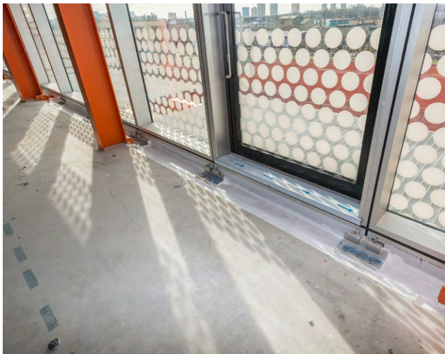
SoftSeal installed as a linear joint seal
