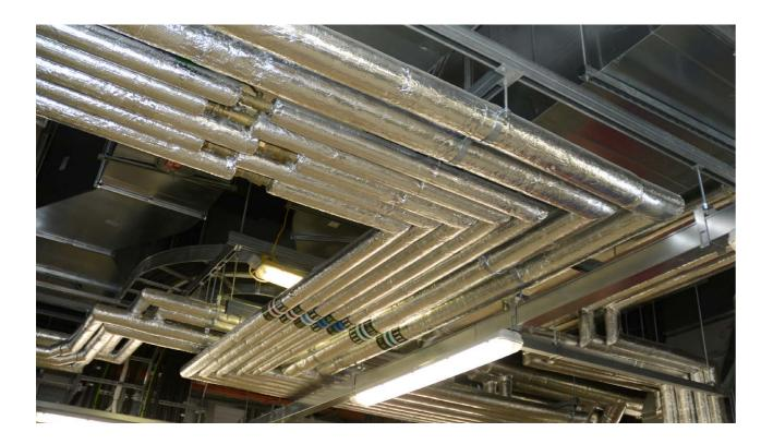
ROCKWOOL HVAC stone wool products offer high performance against a range of criteria; controlling heat gain, minimising heat loss, reducing noise and delivering excellent fire resistance into, and out of the HVAC system, creating safe and healthy working and living environments.
